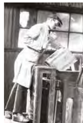
A worker emptying a box of TNT. Note the overshoes to prevent any nails in his boots from causing a spark (source: IST archive)
