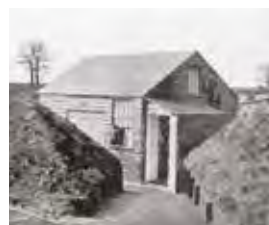
Described by Tilden (1917) 6 as part of a "Cotton Powder Works" it shows the safety features used in explosives manufacturing: a small, lightly constructed building surrounded by earth mounds to deflect any blast upwards
