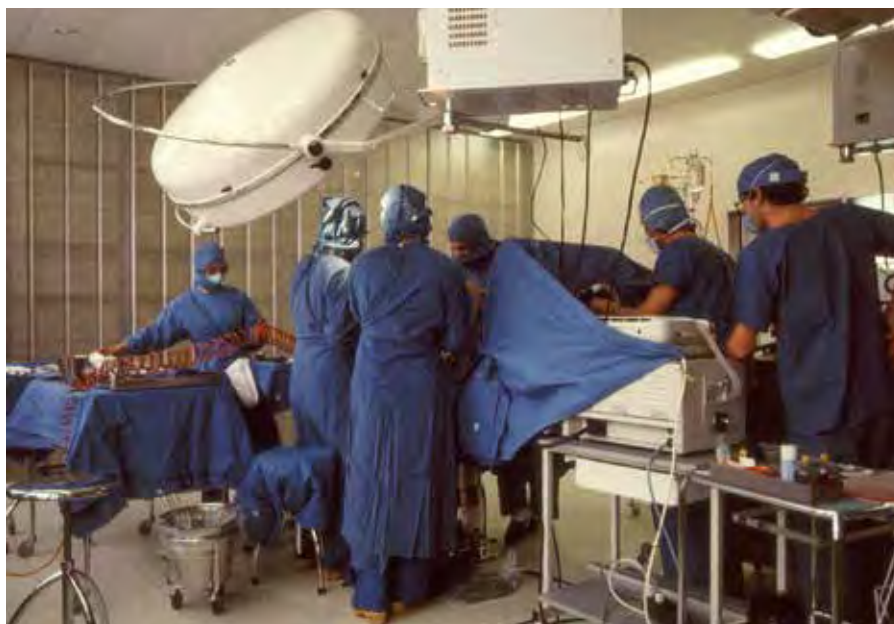
Figure 6: Operating theatre for orthopaedic surgery with horizontal unidirectional airflow, circa 1973 (image courtesy of Schicht Hans H.: 40 years of cleanroom technology - some historical remarks. In: Proceedings of the 17th International Symposium on Contamination Control, Bonn/Germany, 6-9 Sept. 2004, p. 1-10. Edited by: Verein Deutscher Ingenieure (Association of German Engineers), Düsseldorf/Germany (2004))
