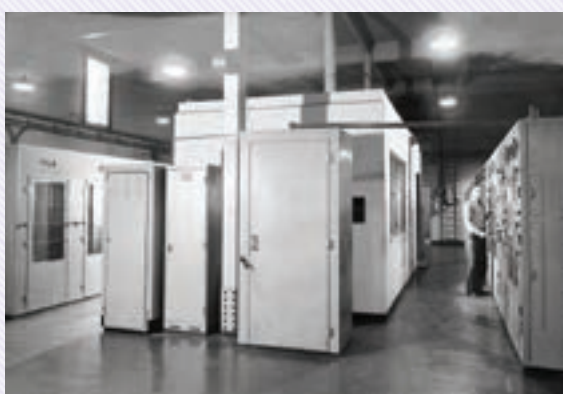
Sender 61, Marconi 100kW SWB18, 1980s and SWB tuning truck, 1980s. Photos copyright Russell W. Barnes
