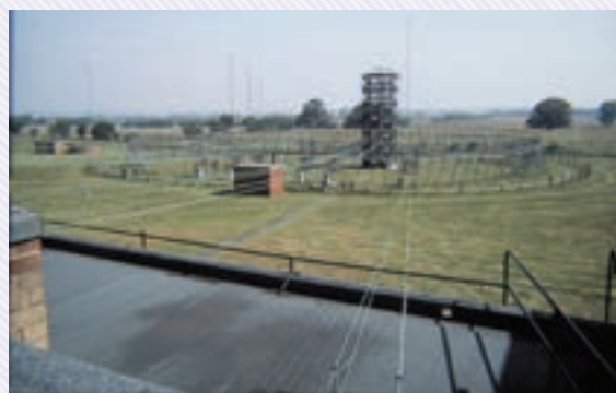
Skelton B (OSE9) aerial switching tower and open wire feeders. Copyright R. W. Barnes
