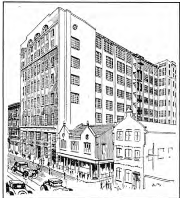
The Post Office’s automatic telephone exchange on Chapel Street, Salford. Building work was completed in 1928 and installation of equipment begun. (Courtesy of Sue Richardson)
